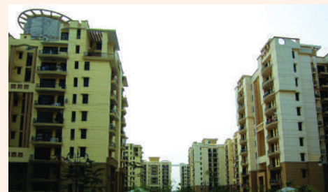
PURVANCHAL SILVER CITY I Sector- 93, Noida (INDIA) TOTAL BUILT-UP AREA SQM 96540 | SQ. FT. 1039160 RESIDENTIAL
