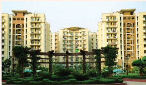
PURVANCHAL SILVER CITY II Sector Pi II, Greater Noida (INDIA) TOTAL BUILT-UP AREA SQM 124835 | SQ. FT. 1343720 RESIDENTIAL
